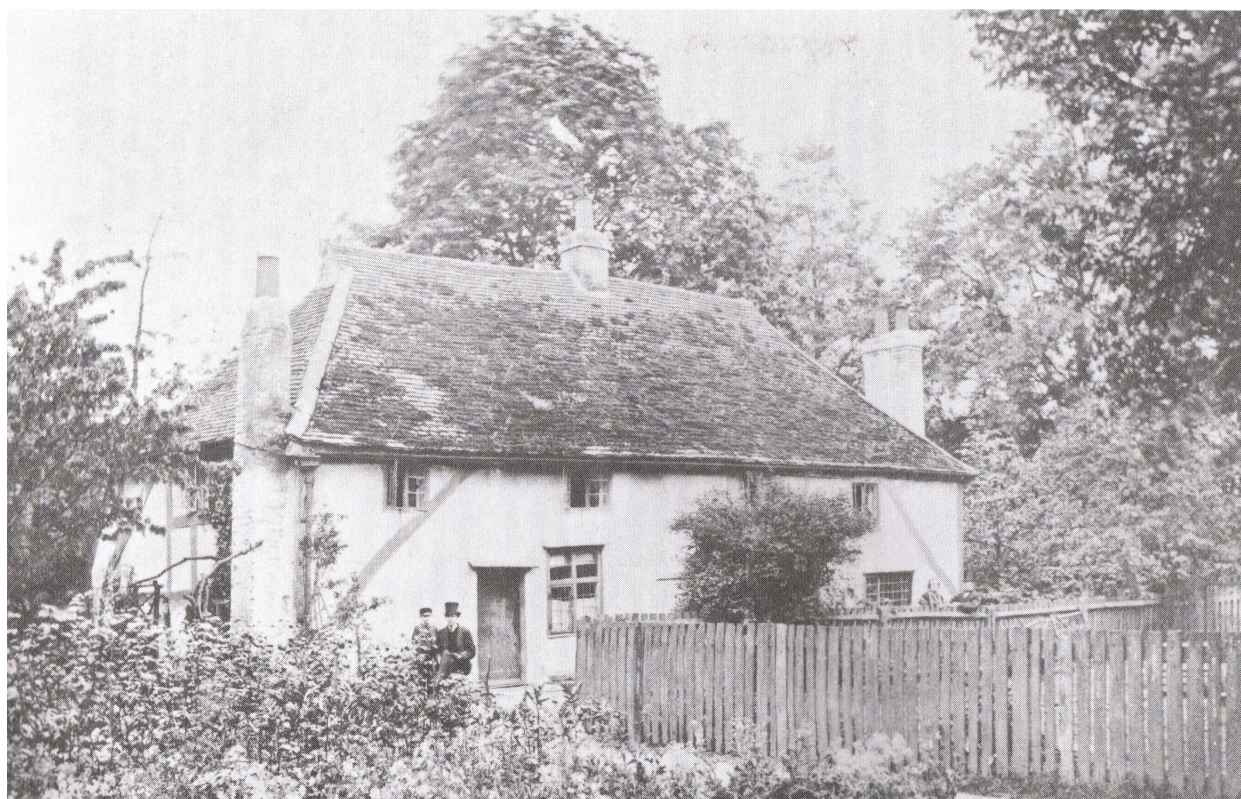
"The Steward's House, Beckenham Lodge Farm circa 1875. Site of the present Church"
